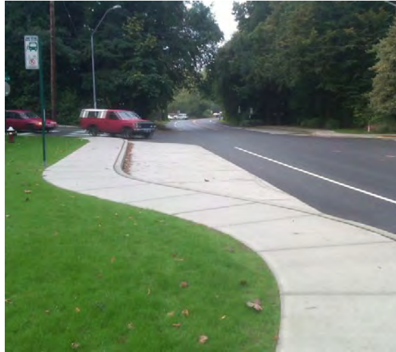
Concrete Bus Pullout
